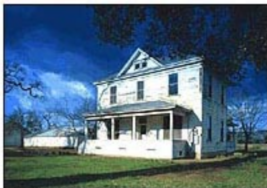
The Sullenger home, which dates to the 1880s, will be restored as part of the Nickel & Nickel winery construction.
